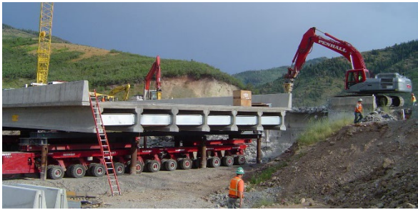
Figure C1.5.1.2.4-2—Method B Support Moments—Single Span Bridges
