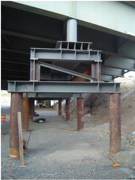
Figure C1.5.1.2.4-3—Method B Support Construction
