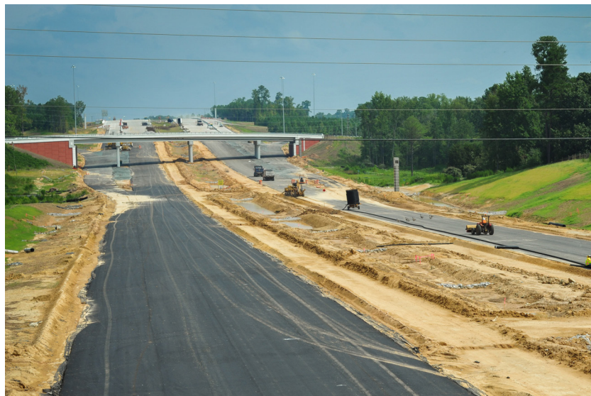
Figure 2-1. Construction Phase—Triangle Expressway (NCTA). Photo courtesy of the North Carolina DOT.
