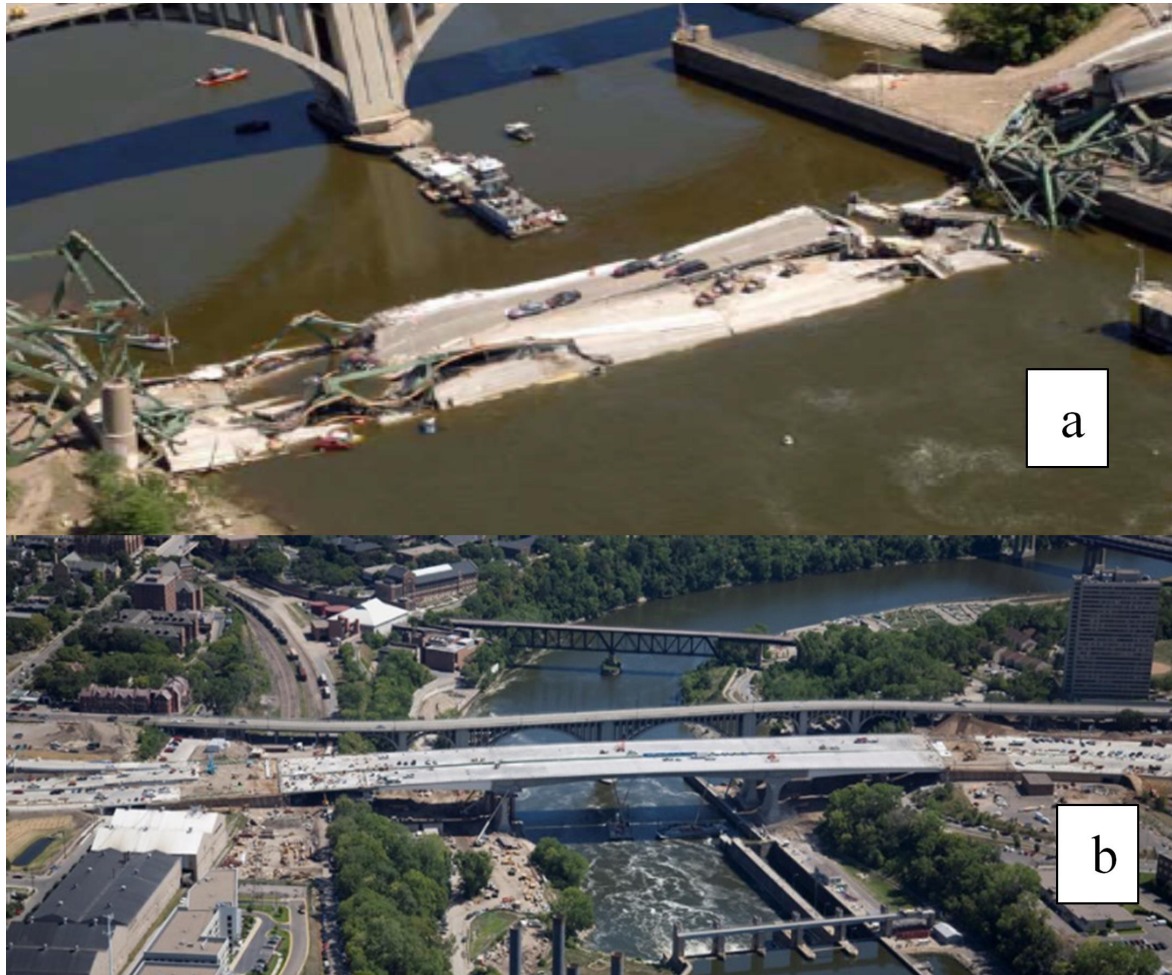
Figure 4-3. I-35W St. Anthony Falls Bridge Before (a) and After (b)
