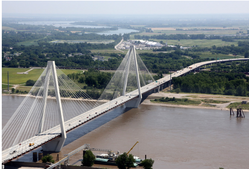
Figure 2-3. Stan Musial Veterans Memorial Bridge. Photo courtesy of the Illinois DOT.
