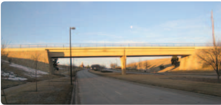
Figure 2-8 This community entry is in a depressed roadway section and passes under a bridge. The use of massive abutments combines with the roadway side slopes to form a gateway. Meadows Parkway Railroad Overpass, Castle Rock, Colorado.
