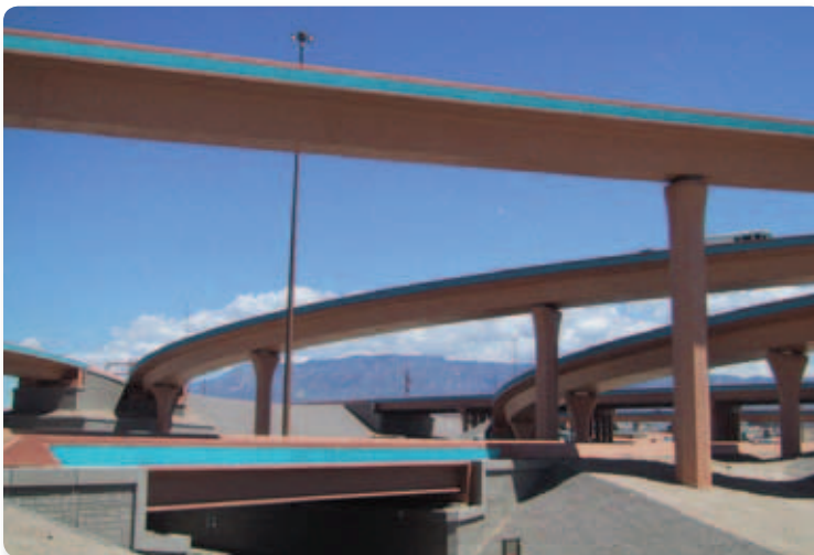
Figure 2-9 Albuquerque's Big I interchange has a theme covering MSE walls, standard details, and colors, developed with community input.
