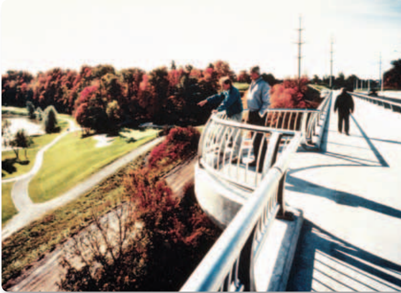
Figure 2-4 Having pedestrians on a bridge suggests the addition of overlooks. Upper Middle Road over 16 Mile Creek, Oakville, Ontario.
