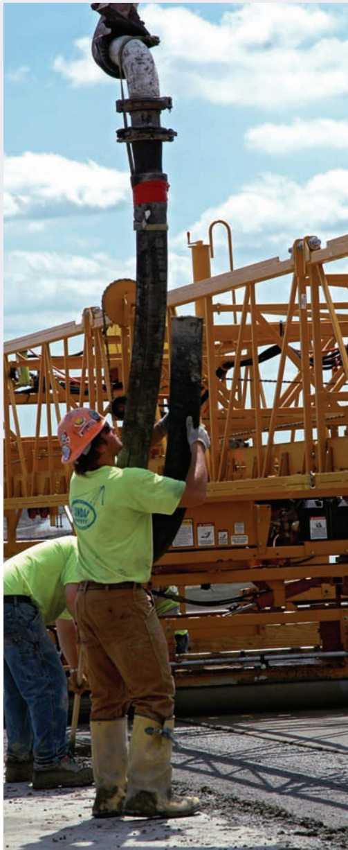
Workers operate concrete pump in the building of the I-94 Business loop of Memorial Bridge North Dakota. Photo courtesy of Mike Kopp, North Dakota Department of Transportation, 2008.
