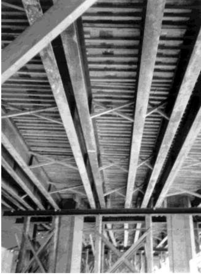
Figure 2.3.1-1—Wood Cross-Bracing Between Longitudinal Stringers
