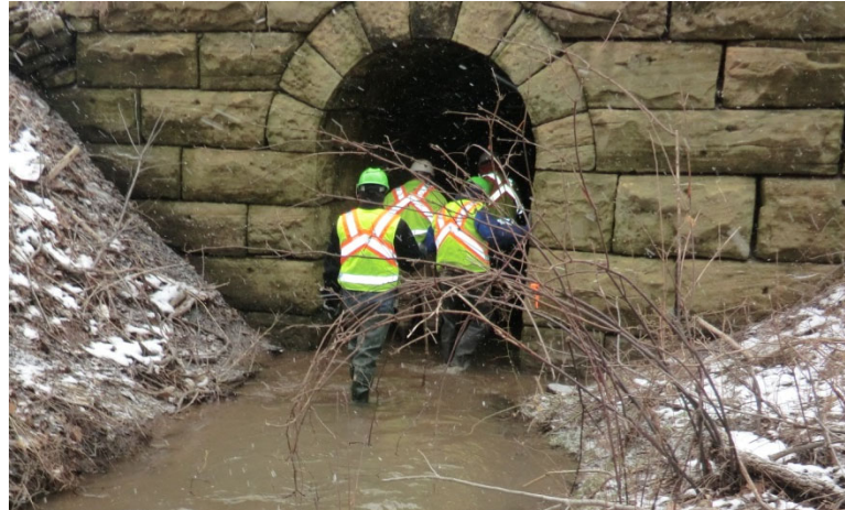
Figure 3.6.1-1—Person-entry Inspection of a Masonry Culvert (Photo courtesy of Ohio Department of Transportation)
