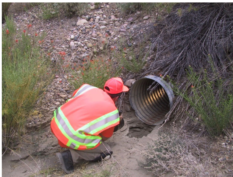
Figure 3.6.2-1—Non-entry Inspection of a Corrugated Metal Culvert
