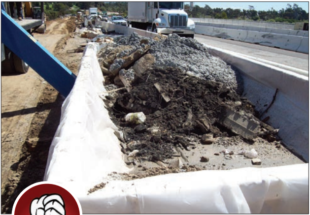
Fig. 2-9. While there appears room in this concrete washout, it has reached the recommended 75 percent capacity and should be cleaned out. Source: RBF Consulting
