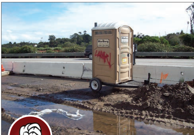
Fig. 2-10. This sanitary facility has not been provided with secondary containment, and is located very close to a large amount of concentrated drainage.
