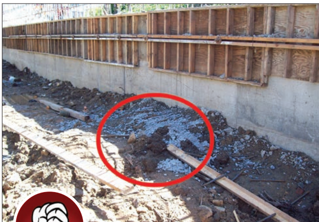
Fig. 2-14. This picture depicts residue from cleanout of a concrete truck not performed in a controlled washout area.
