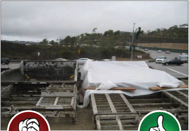
Fig. 2-8. Left—A concrete washout left unprotected. Source: Nevada DOT
