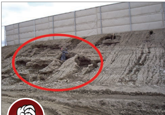
Fig. 1-5. All forms of erosion can occur at a construction site. Here the rills and gullies will need repair and could have been prevented with proper BMPs. Source: RBF Consulting
