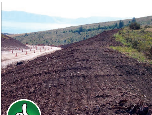
Fig. 2-4. Track walking is among the most common techniques used to roughen a slope. Grooves should be created parallel to the slope contour line.
