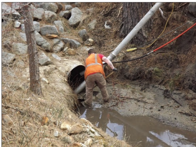
Fig. 2-1. Crews clean a culvert.
