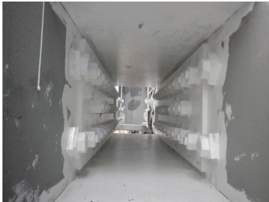
Figure 2-3—Truss bottom chord field splice (inside view)
