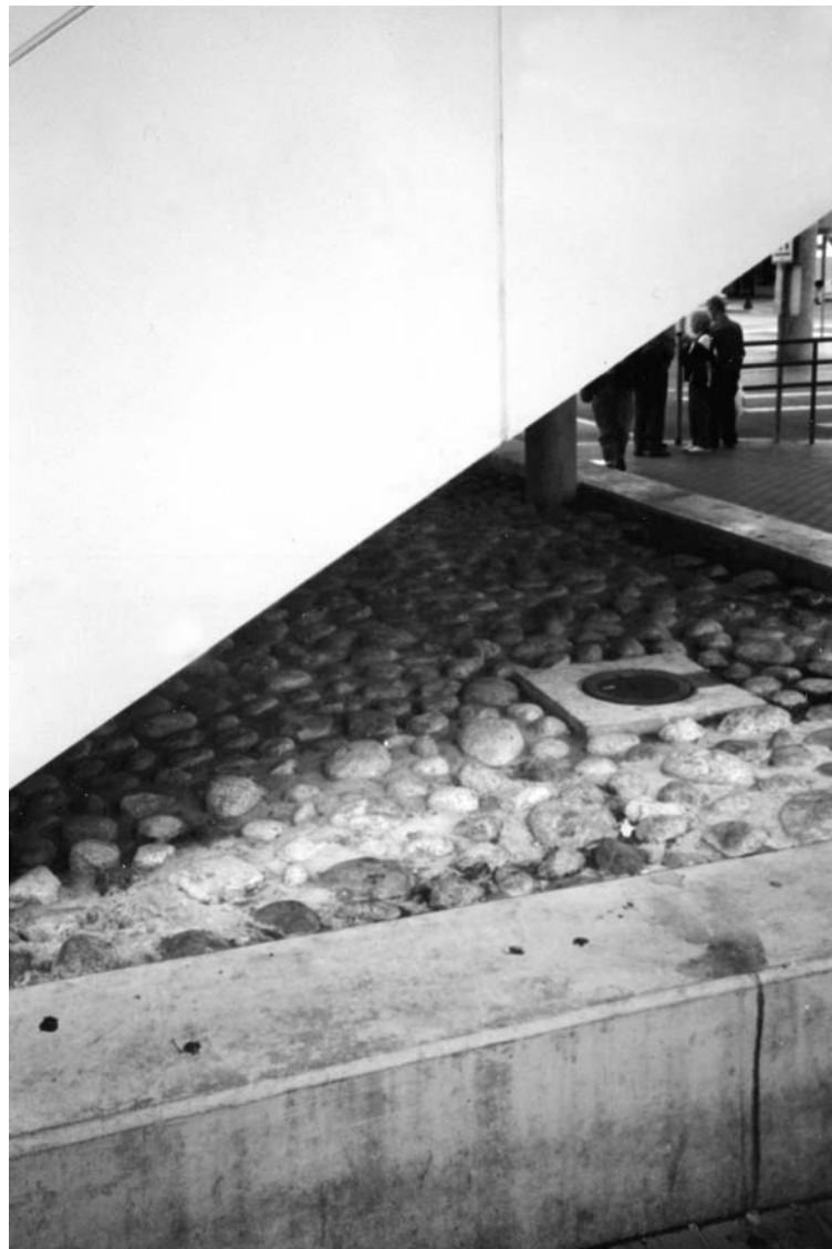
FIGURE 3-5. River stone embedded in concrete beneath low overhang discourages vagrancy. BC Transit, Vancouver, British Columbia, Canada.
