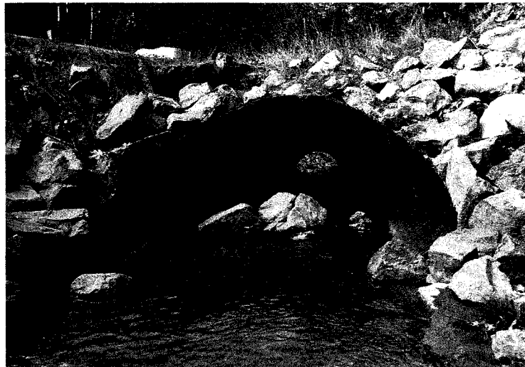
Figure III-3. Example of countersunk culvert.
