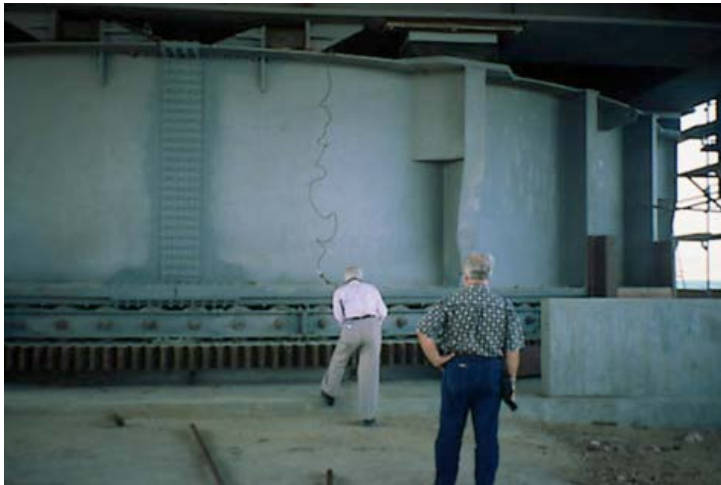
Figure 1.3.2.1-6 – Rim bearing swing-span rollers and rack
