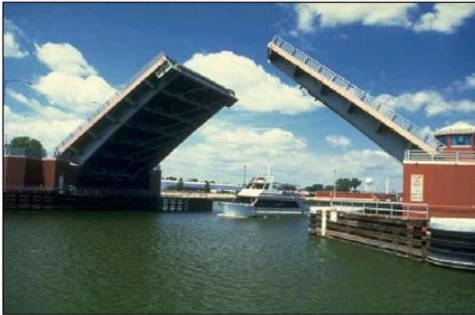
Figure 1.3.1.1-1 – Double-leaf bascule bridge
