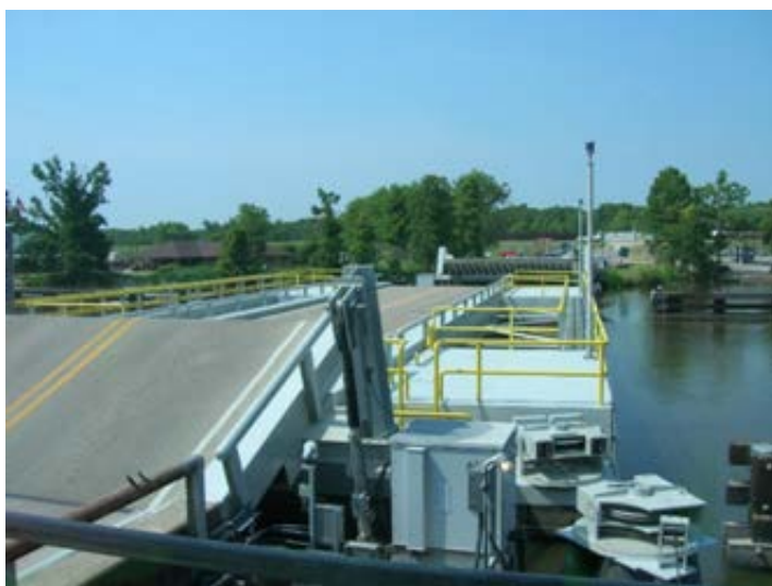
Figure 1.3.4-1 – Pontoon swing-span bridge with wire rope operation, Louisiana
