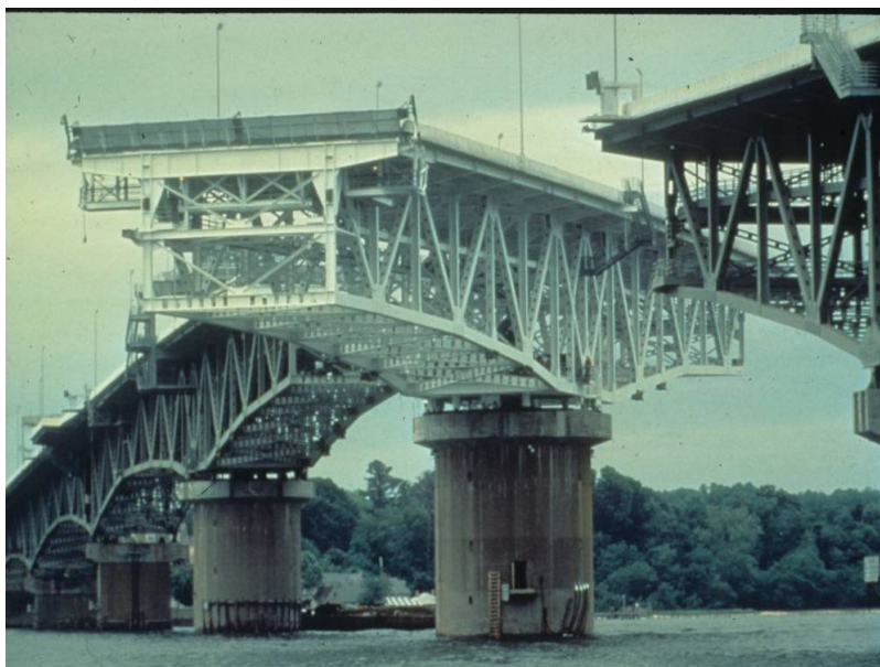
Figure 1.3.2-1 – Swing-span bridge
