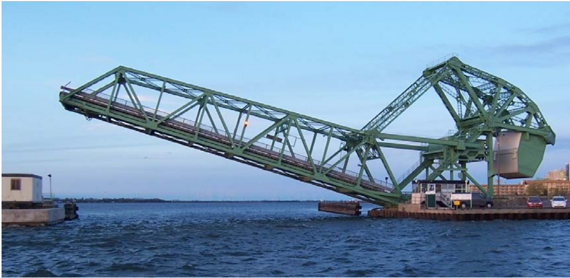
Figure 1.3.1.1-7 – Heel-trunnion (Strauss) type bascule bridge
