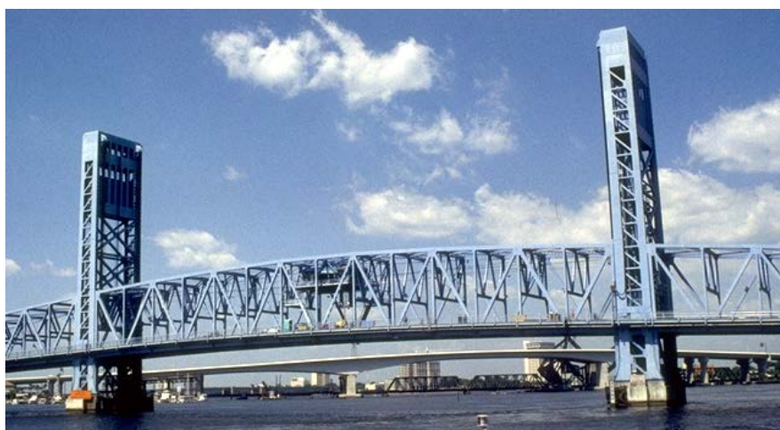
Figure 1.3.3.1-3 – Span-drive vertical-lift bridge
