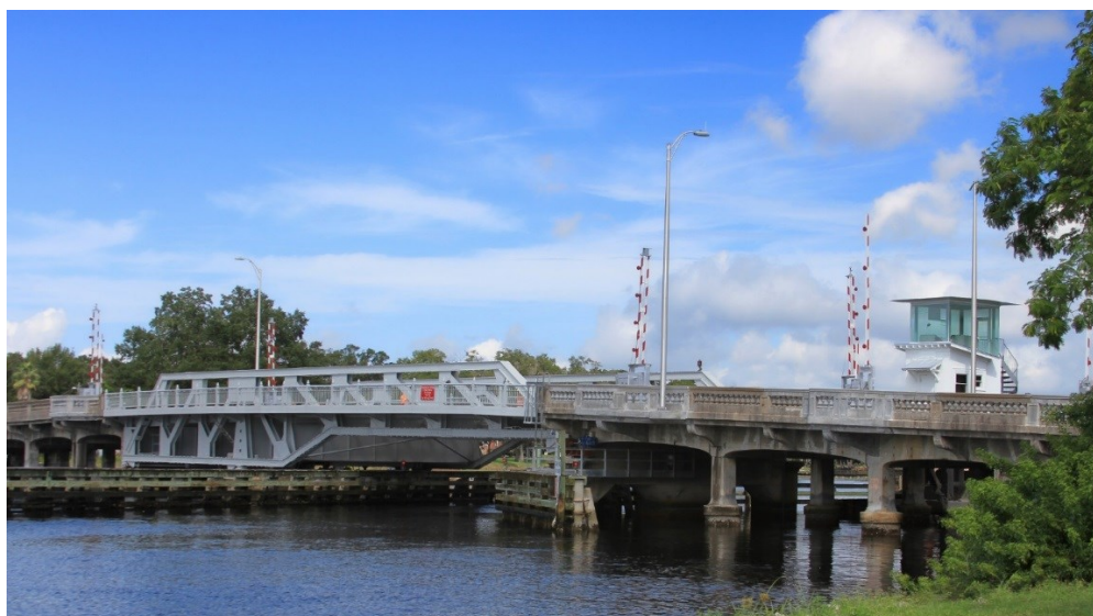
Figure 1.3.2-2 – Bob-tail swing-span bridge
