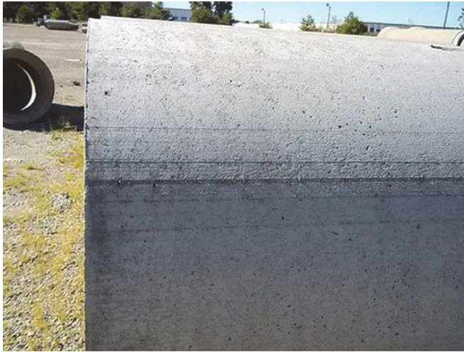
Figure 7 —Acceptable Lines Caused by Form Jacket during Stripping ( Photo Courtesy of ACPA )
