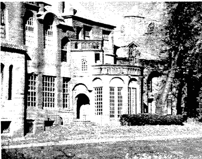
Fig. 1.5—Note the abundance of windows of widely differing styles. The house was wired for electricity at the time of construction but Mercer preferred kerosene and oil lamps. The windows were so arranged to direct daylight into specific corners, or down a hallway, wherever deemed necessary.
