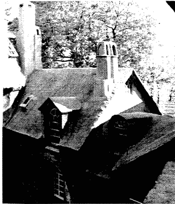
Fig. 1.6—Of the three Mercer buildings his home is the favorite of many visitors because it is the most personal. The remarkable structure actually envelops a small 18th century farmhouse, literally encasing it with concrete. This slide shows that portion of Fonthill.
