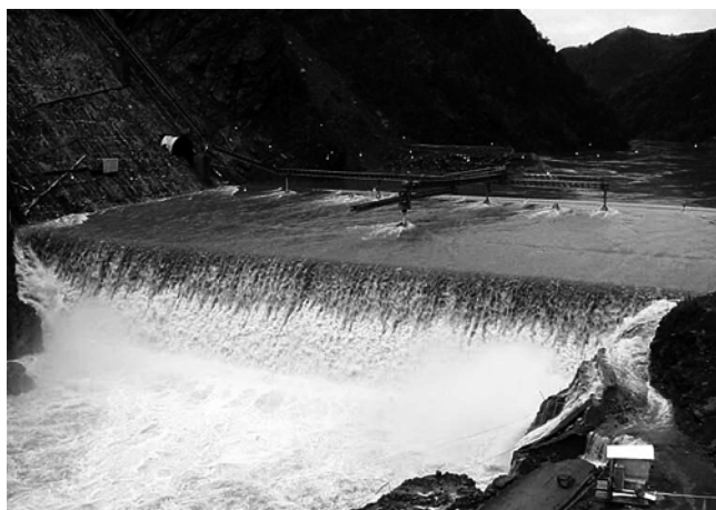
Fig. 1.11—Le Presa Ralco Dam, Chile, overtopping during construction. (Photo courtesy of B. Forbes and E. Warren, 2003).
