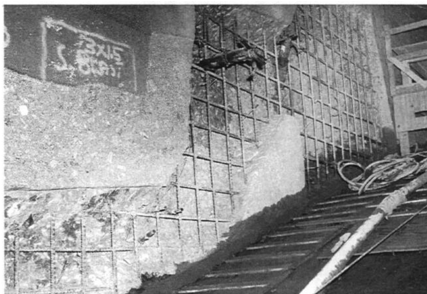
Fig. 2.2-Dworshak Dam. Extent of outlet surface preparation prior to concrete and mortar placements
