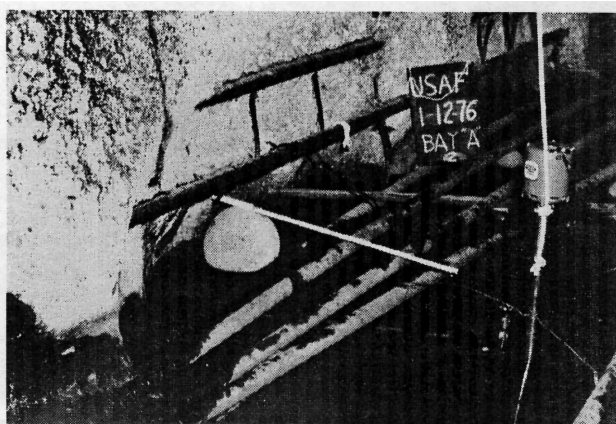
Fig. 3.6-Abrasion erosion damage to discharge lateral: Upper St. Anthony Falls Lock
