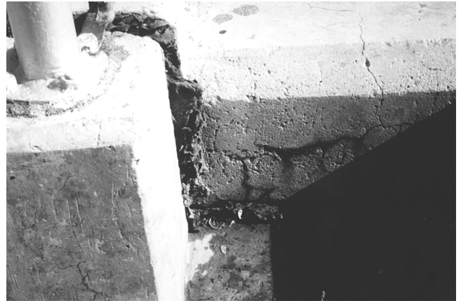
Fig. 5—Photograph showing closure of a joint and extrusion of joint-filling material due to ASR expansion.
