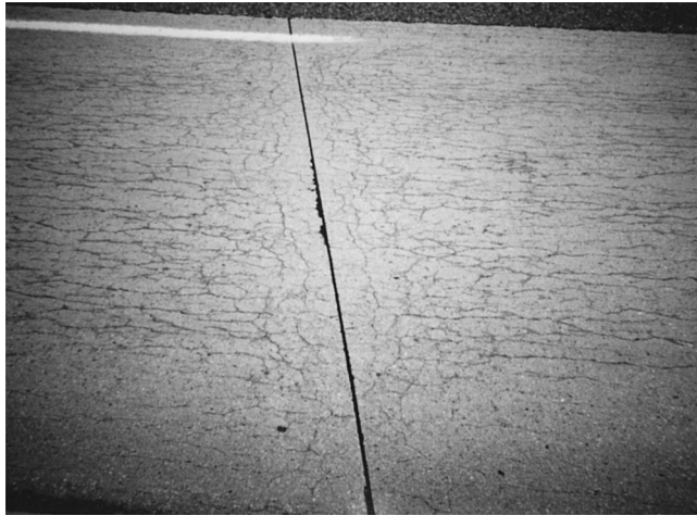
Fig. 4—Photograph of pavement affected by ASR. Typical longitudinal cracking is parallel to the slab free edges, with additional transverse cracks in the areas near the transverse joints.
