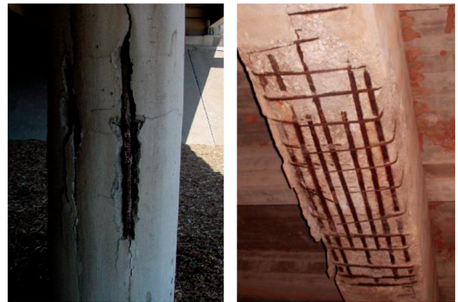
Fig. 4.1—(a) Damaged bridge column and (b) damaged bridge beam as a result of reinforcement corrosion (photos courtesy of D. Trejo).
