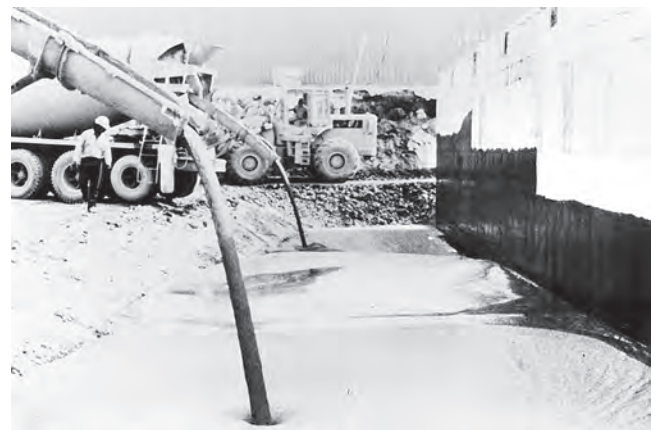
Fig. 3.2a—Using CLSM to backfill adjacent to building foundation wall.
