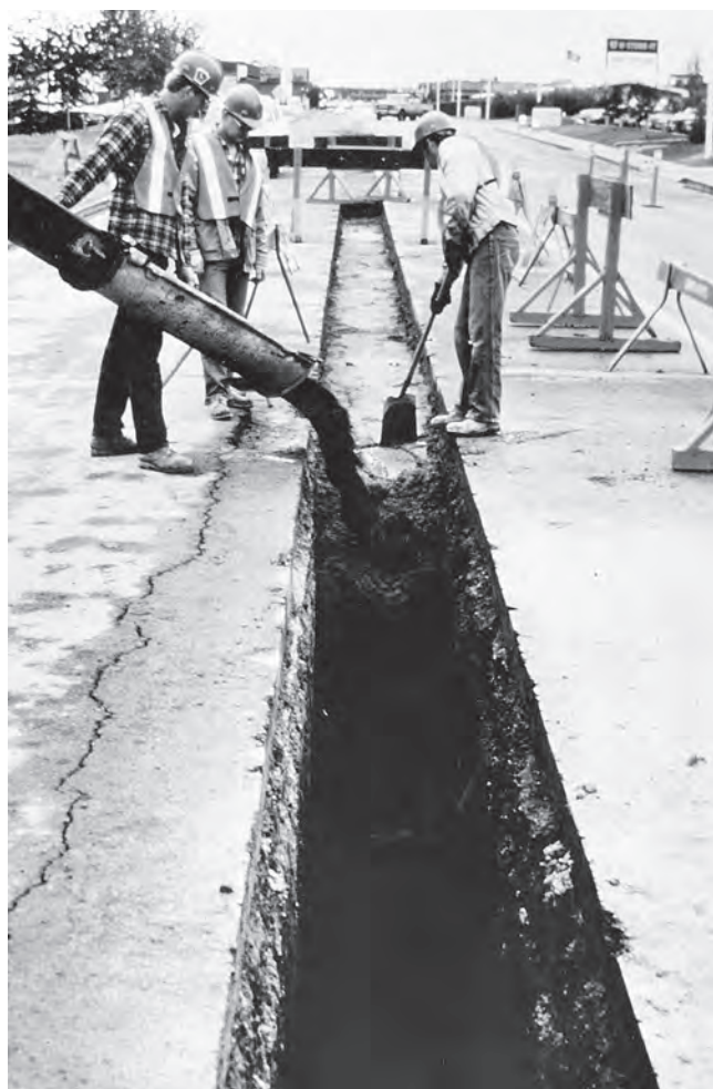
Fig 3.2b—Backfilling utility cut with CLSM.
