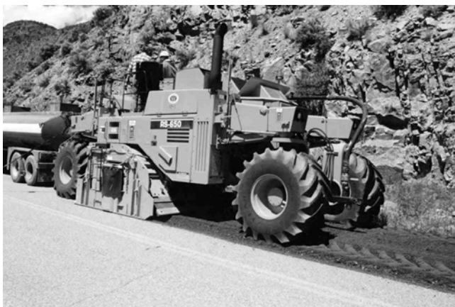
Fig. 3.2—Complete pulverization of asphalt and base.
