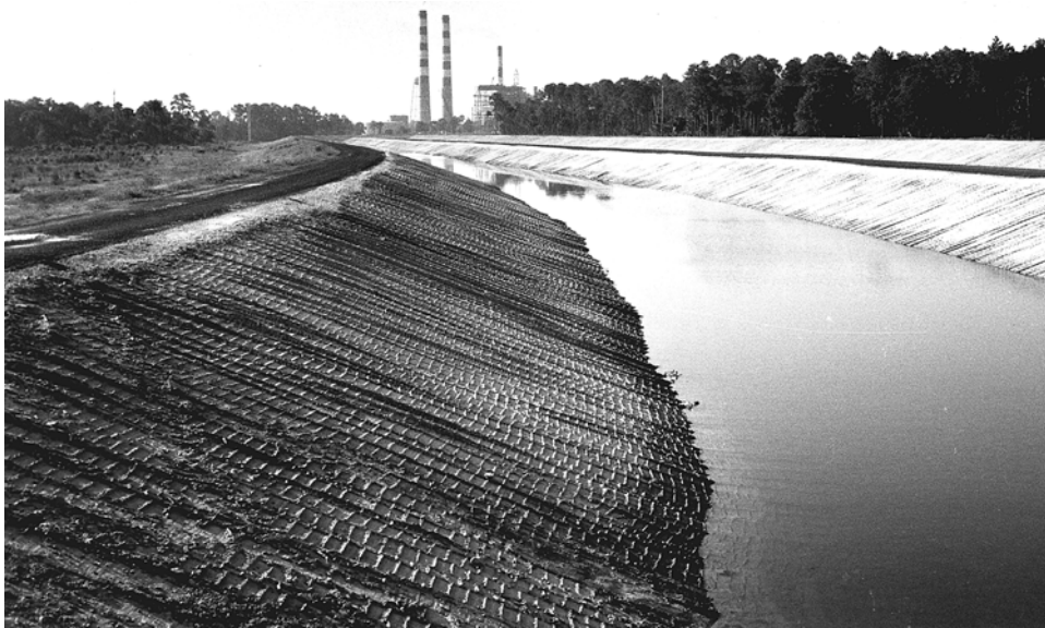
Fig. 3.7—Soil cement slope plating for cooling water flume at Florida power plant.
