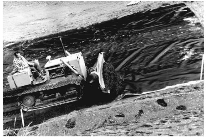
Fig. 3.9—Spreading soil cement on membrane at 3:1 slope Apalachin, NY.
