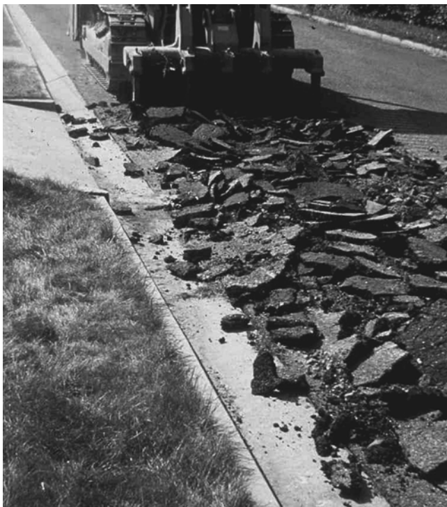
Fig. 3.1—Initial pulverization of asphalt surface and base.
