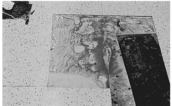
Fig. 1.4—Adhesive degradation leading to debonded solid vinyl tile installed over asbestos tile. (Courtesy of Peter Craig.)
