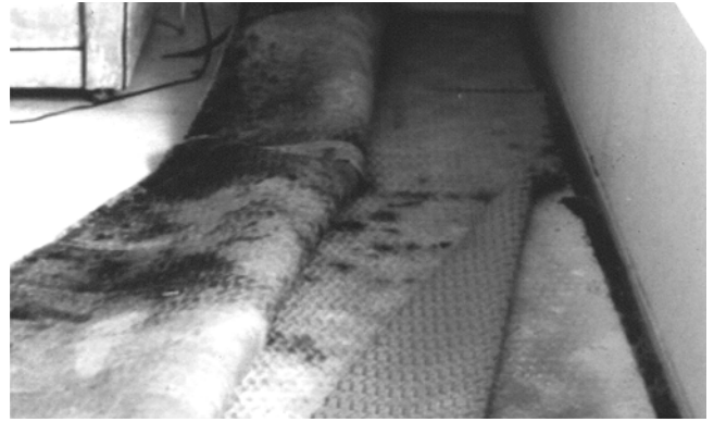
Fig. 1.3—Mold growth in carpet due to moisture in concrete. (Courtesy of Floor Seal Technology, Inc.)
