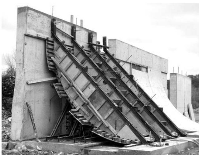
Fig. 3.5.4.a—Full-scale preconstruction mockup used for the Contemporary Arts Center, Cincinnati, OH.
