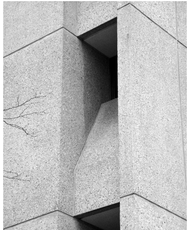
Fig. 3.2.3—Architectural cast-in-place wall with precast window spandrels to match.
