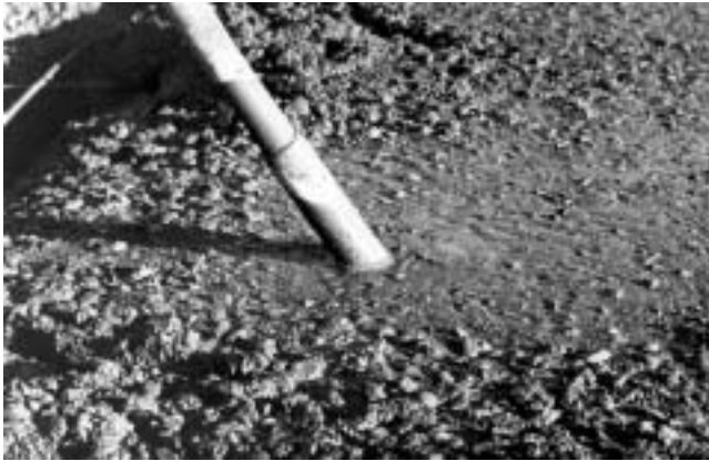
Fig. 4.1—Internal vibratory “liquefying” low-slump concrete.
