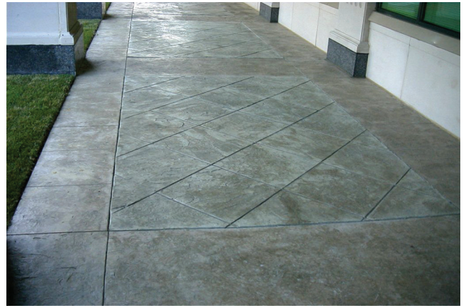
Fig. 4.3a—Color hardeners are often used in combination with texturing techniques such as stamping (courtesy of Patterned Concrete of Pennsylvania Inc.).
