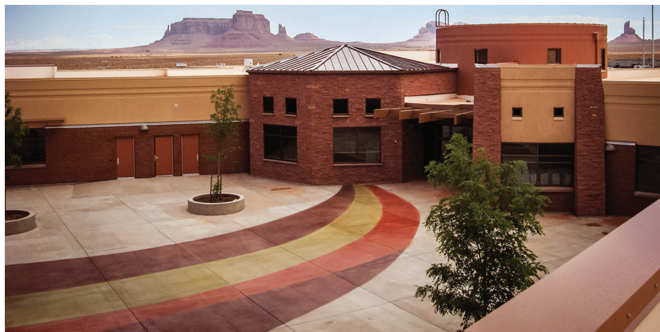
Fig. 1.2b—Decorative concrete applications such as post placement colorant or staining complement or enhance the overall aesthetics of a project (courtesy of PROSOCO).
