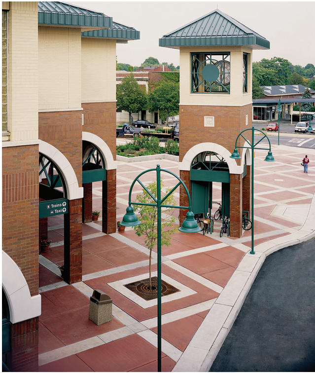
Fig. 3.2.1—Good communication ensures the design intent is achieved (courtesy of L. M. Scofield Company).
