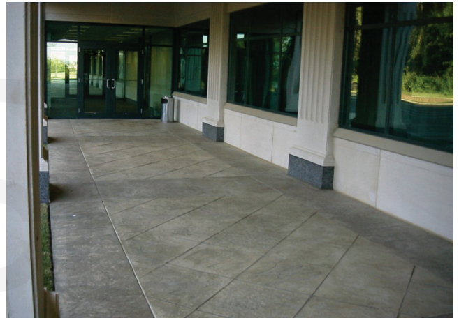
Fig. 4.3b—Color hardeners are often used in combination with texturing techniques such as stamping (courtesy of Patterned Concrete of Pennsylvania Inc.).
