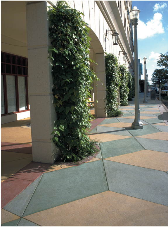
Fig. 4.2.3—Integrally colored concrete places with alternating sections delineated by construction joints (courtesy of L. M. Scofield Company).
