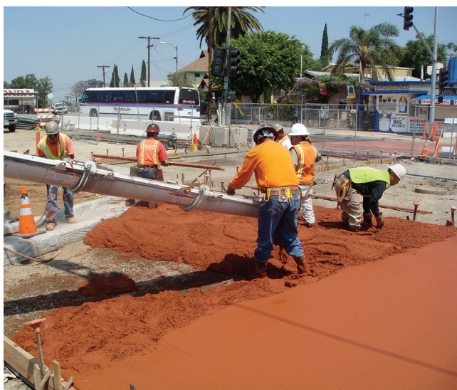
Fig 4.2.1b—Integrally colored concrete is batched and placed like uncolored concrete (courtesy of Davis Colors).
