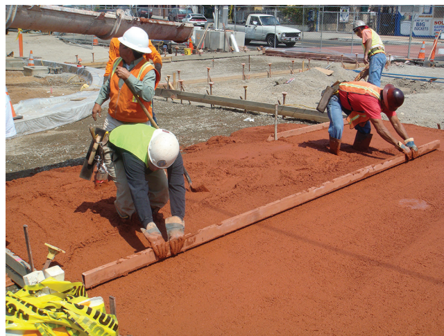
Fig. 4.2.1c—Integrally colored concrete is placed using standard practices (courtesy of Davis Colors).
