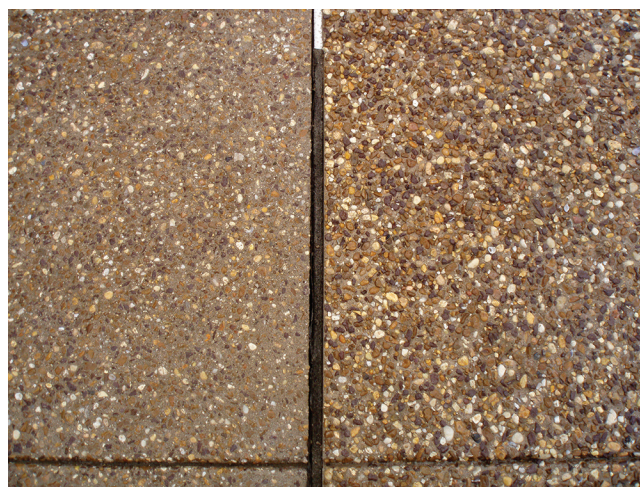
Fig. 4.4.1—Examples of exposed aggregate achieved on identical slabs with surface retarders rated for different exposure levels (courtesy of Nick Sorrentino).
