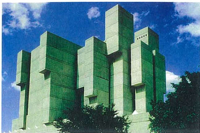
Fig. 1.4—Building design accented with horizontal joints; quality construction provides a highly functional and aesthetic workplace.
