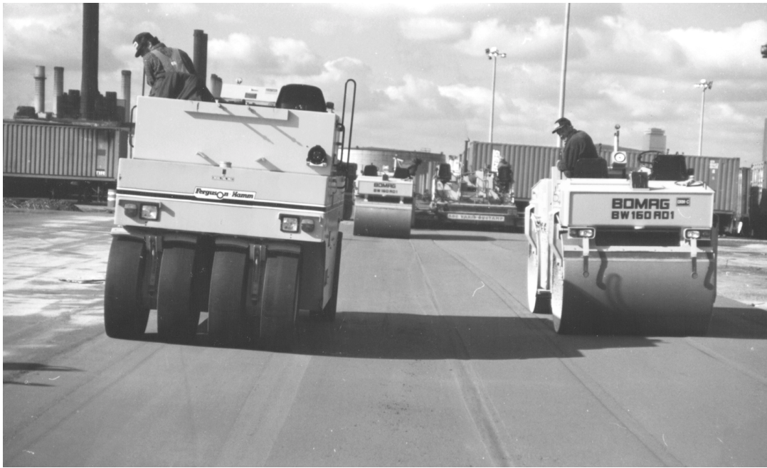
Fig. 2.3—Rubber-tired roller compaction
