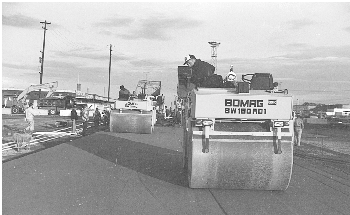
Fig. 2.2—Vibratory roller compaction
