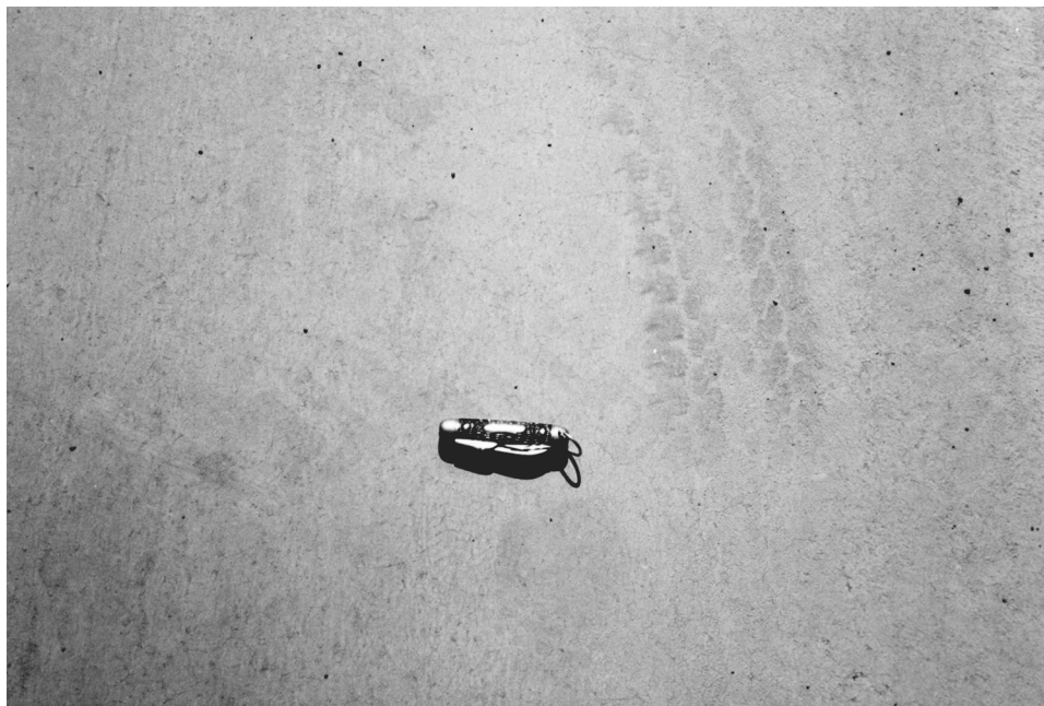
Fig. 2.8—Excellent RCC pavement surface — Ft. Bliss, Texas
