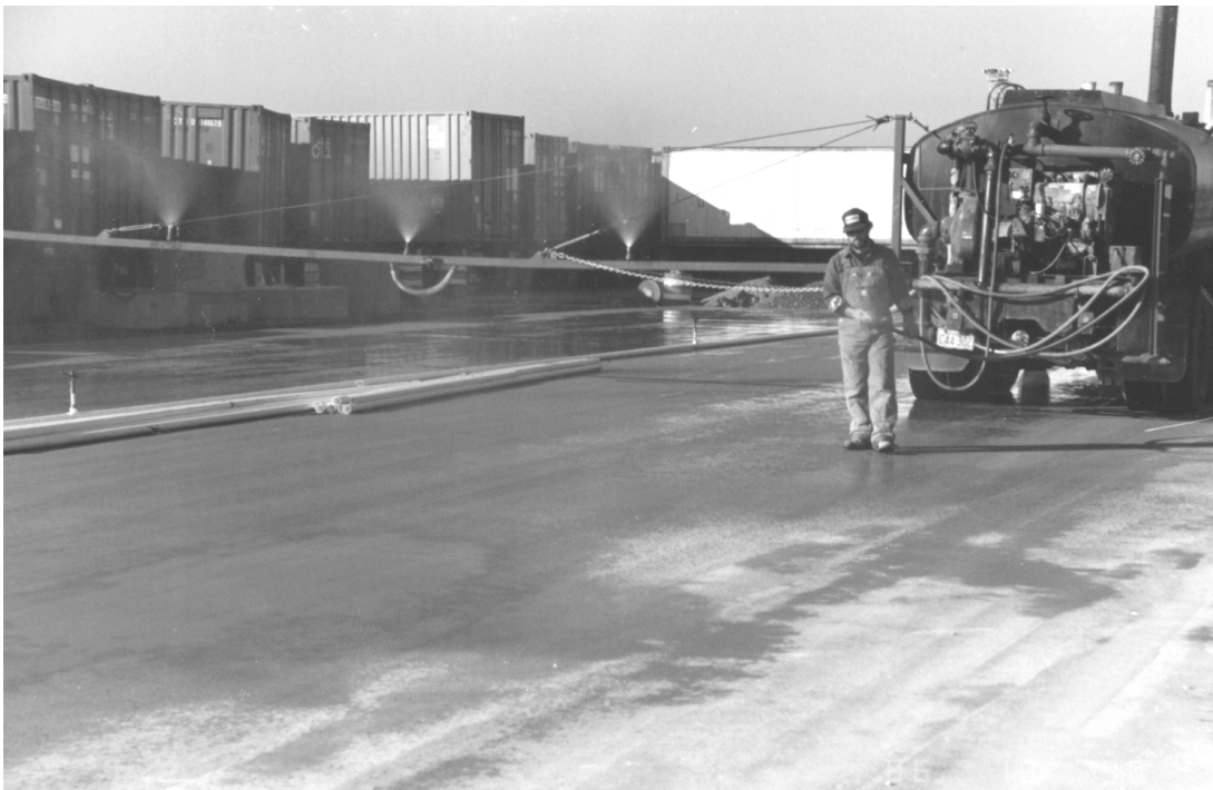
Fig. 2.4—Fog curing of freshly placed RCC pavement
