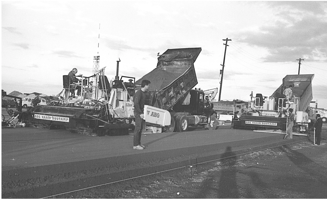
Fig. 2.1—RCC placement using modified asphalt pavers
