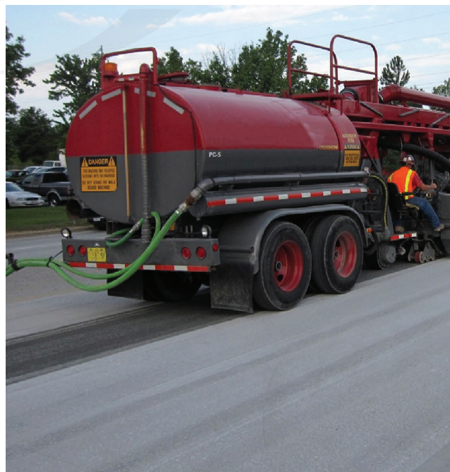
Fig. 3.3e—Diamond grinding of RCC provides for a smooth and quiet surface. Diamond ground section is behind vehicle.
