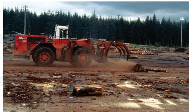
Fig. 4.8—RCC pavement constructed at a log handling facility (Harrington et al. 2010).
