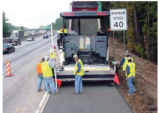
Fig. 4.6—Example of RCC used to reconstruct shoulders on I-285 near Atlanta, GA (Harrington et al. 2010).
