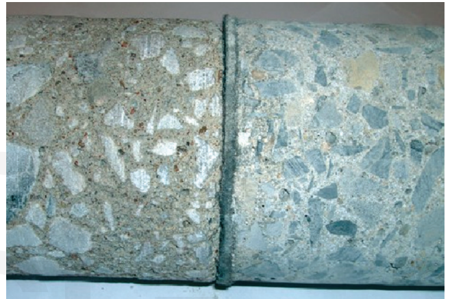
Fig. 4.3.1—Pavement cores showing multilayer system with geotextile fabric layer (Harrington et al. 2010).
