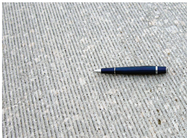
Fig. 3.3d—Surface texture of RCC after diamond grinding (Harrington et al. 2010).
