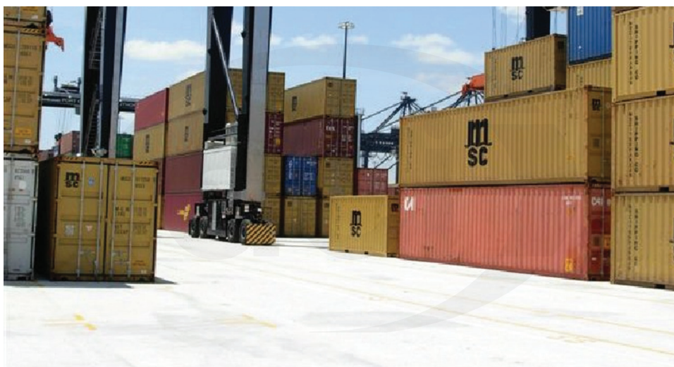
Fig. 4.1—Example of RCC port facility in Houston, TX (Harrington et al. 2010).
