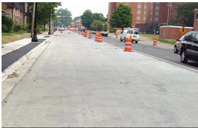
Fig. 4.4—RCC pavement constructed on an arterial street in Columbus, OH (Harrington et al. 2010).
