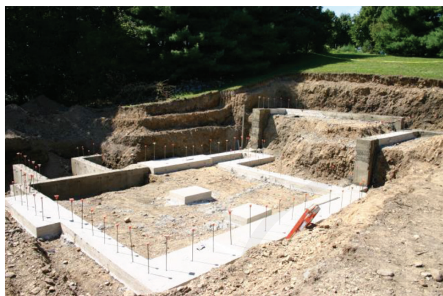
Fig. 4.3.6.2b—Footing with dowels.
