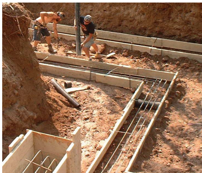
Fig. 4.2.1b—Reinforced footing.
