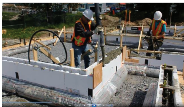
Fig. 4.3.8.1a—ICF stem wall with bag footing being poured concurrently with steel fiber-reinforced concrete.
