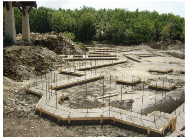
Fig. 4.3.6.1b—Footing with formed keyway.
