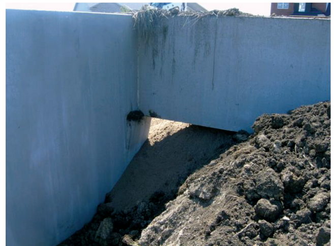
Fig. 4.3.5—Discontinuous footing at a common wall step.
