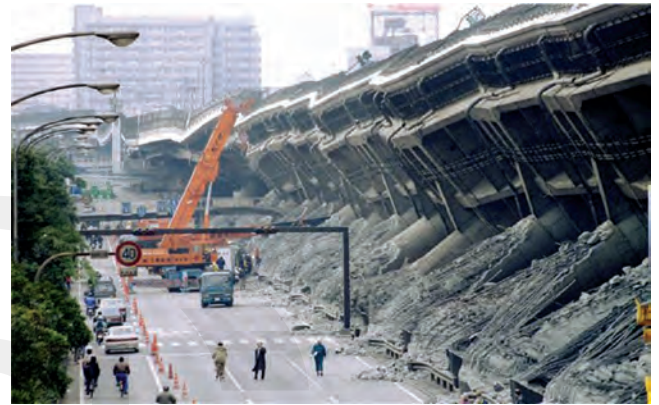
Fig. 1.2c—Arterial bridge in Kobe, Japan, earthquake.
