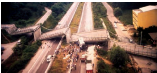
Fig. 1.2.1a—Unseating of bridge spans, Kocaeli earthquake (Turkey) (Erdik 2008).
