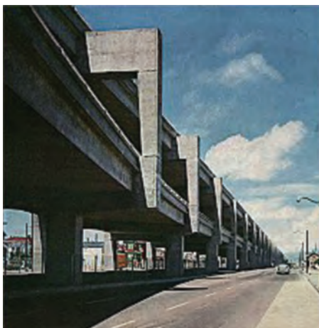
Fig. 1.2.4a—I-880 Cypress double deck viaduct before failure.
