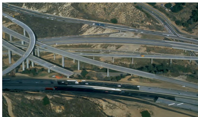
Fig. 1.2.4c—Aerial view of 5/14 Interchange, Los Angeles, CA, 1994 Northridge earthquake (FEMA 2009b).
