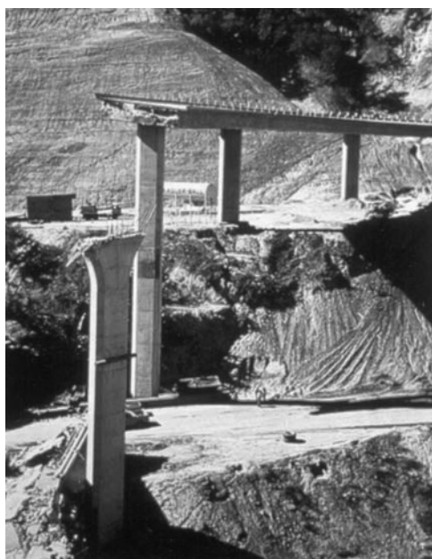
Fig. 2.4—Collapse of a bridge superstructure due to inadequate expansion joint details. (Courtesy of University of California, San Diego.)
