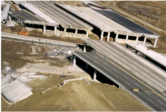
Fig. 4.2.4k—Column failures and loss of seat support, Interstates 5 and 210 in Southern California, 1971 San Fernando Earthquake. (Courtesy of NISEE, University of California, Berkeley, CA [Steinbrugge 1971].)
