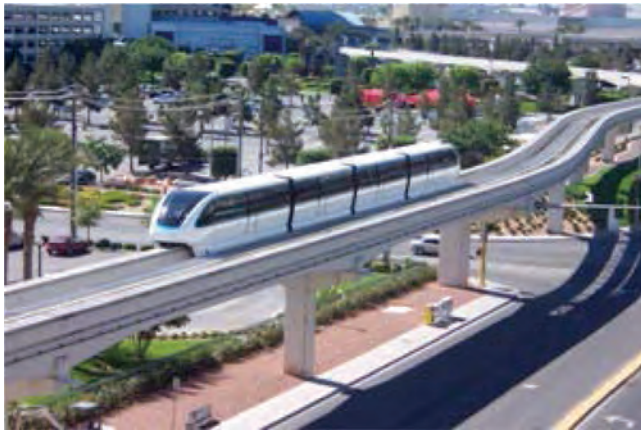
Fig. 3.5.2a—Design decisions to fit guideway around existing features (courtesy of Las Vegas Monorail Co.).
