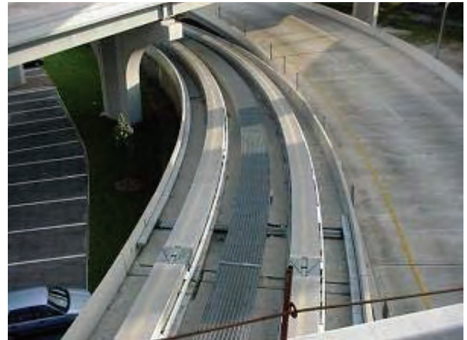
Fig. 3.3.2a—Walkway between rails (courtesy of Jacksonville Transportation Authority).
