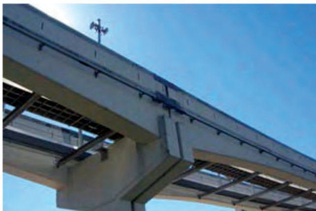
Fig. 3.3.2b—Walkways between rails (courtesy of Las Vegas Monorail Co.).
