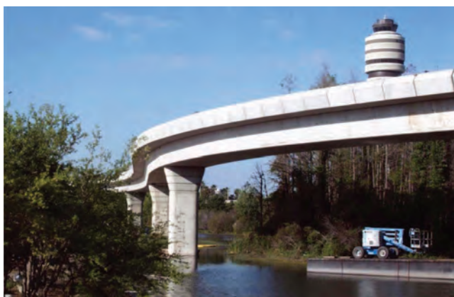
Fig. 3.2.2.1a—Precast box girders for sharp curvature (courtesy of PCA). Continuity has been provided through curved alignment.
