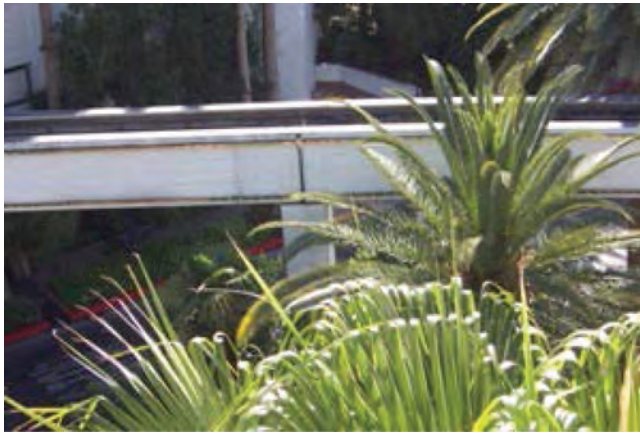
Fig. 3.2.2.1b—Precast concrete girders (courtesy of MGM Mirage, Inc.). Example of simple span construction.
