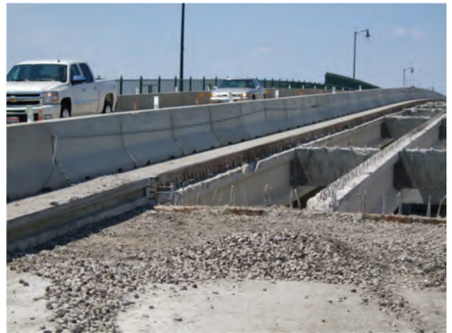
Fig. 3.2.3—Traffic allowed on a bridge during deck slab widening.
