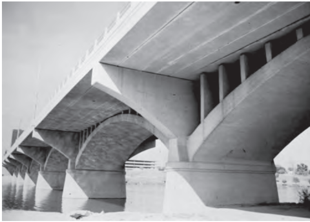
Fig. 3.2.1a—Concrete arch widening with prestressed sections.
