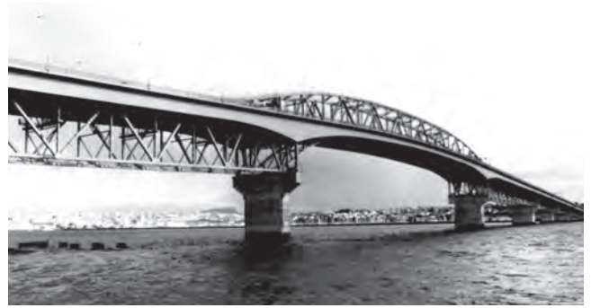
Fig. 3.2.1b—Widened bridge with steel box girders, Auckland Harbor in New Zealand.
