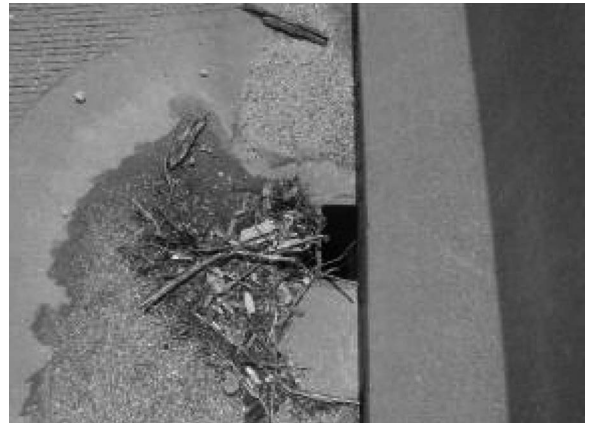
Fig. 3.6.3—Poor design and lack of maintenance permit debris to accumulate and block deck drains.
