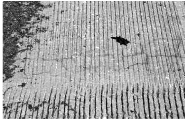
Fig. 3.8(a)—Pattern cracking.
