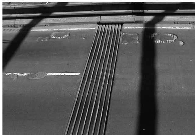
Fig. 3.7.7—Example of modular joint system.
