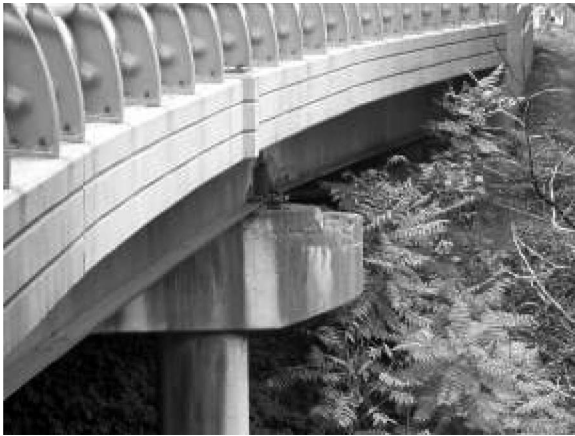
Fig. 3.6.1(b)—Water leakage through failed joint causes corrosion and deterioration of pier cap.
