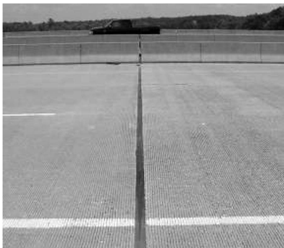
Fig. 3.7.1—Field-molded (pourable) joint seal system.
