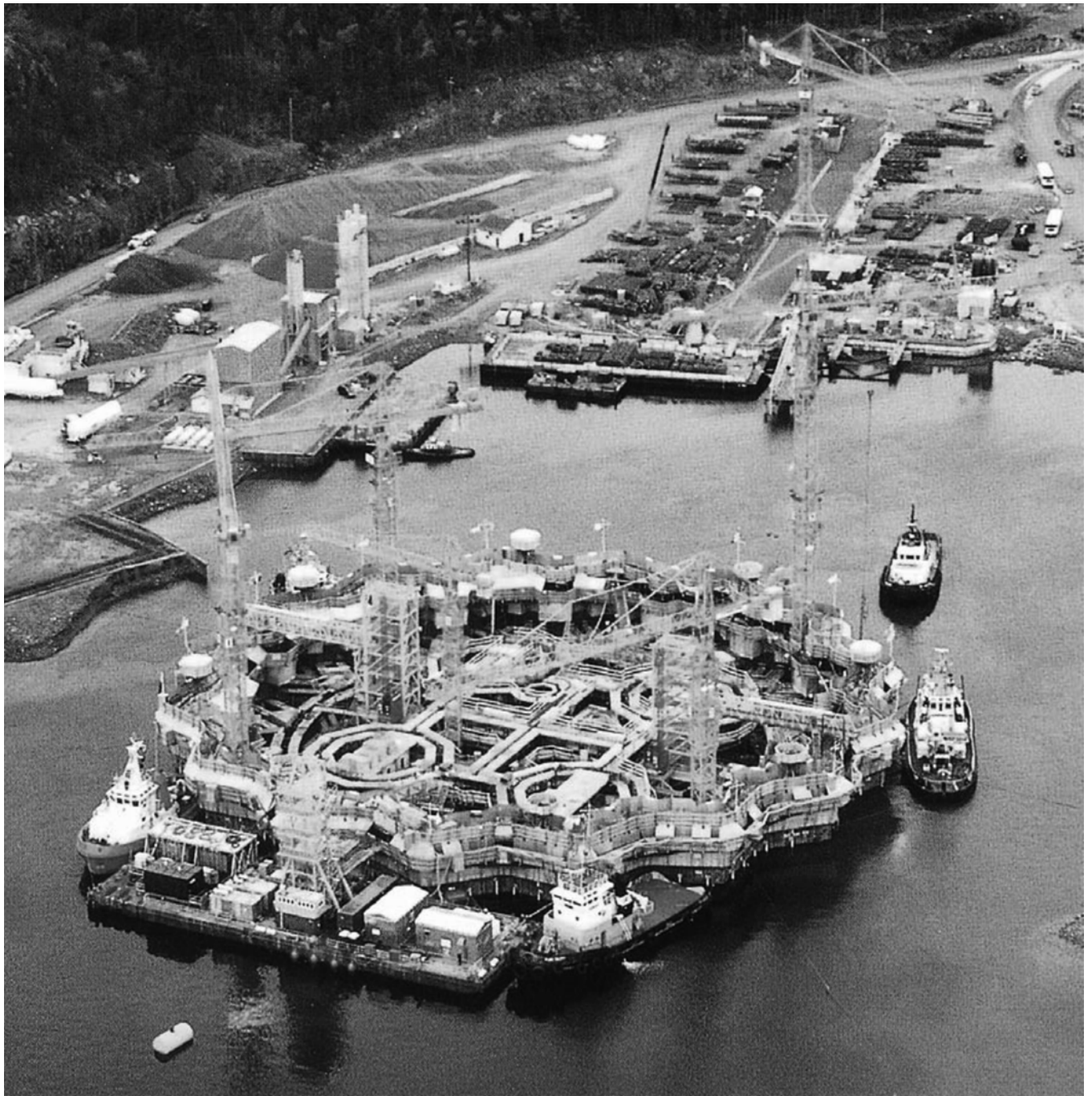
Fig. 3.6—Hibernia offshore GBS under construction.
