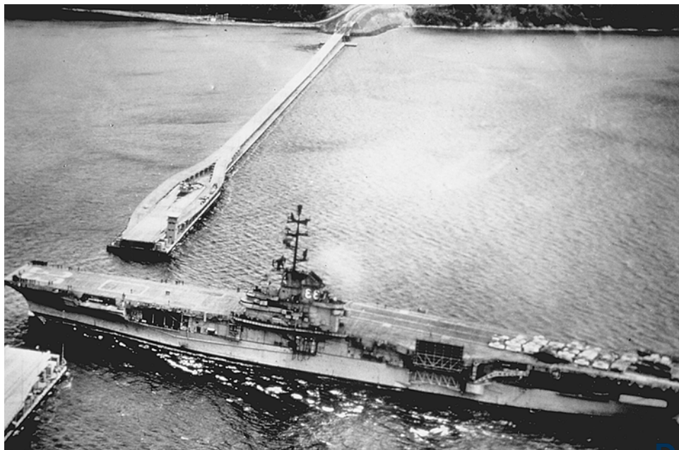
Fig. 3.10—Hood Canal floating bridge.
