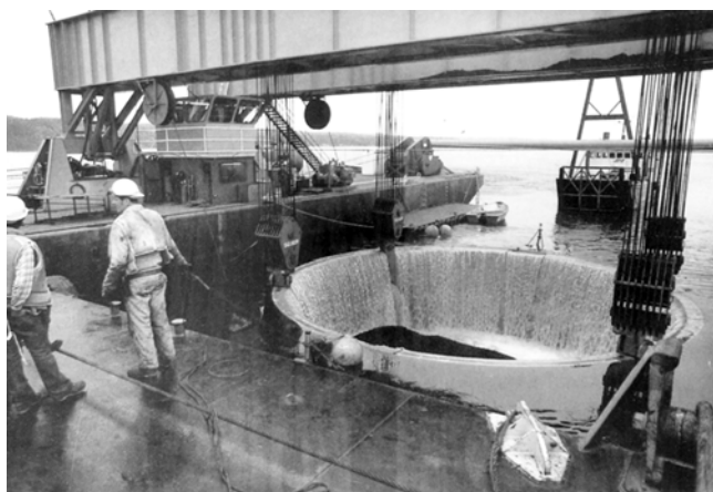
Fig. 3.13—Hood Canal Bridge span replacement concrete gravity anchor during installation.
