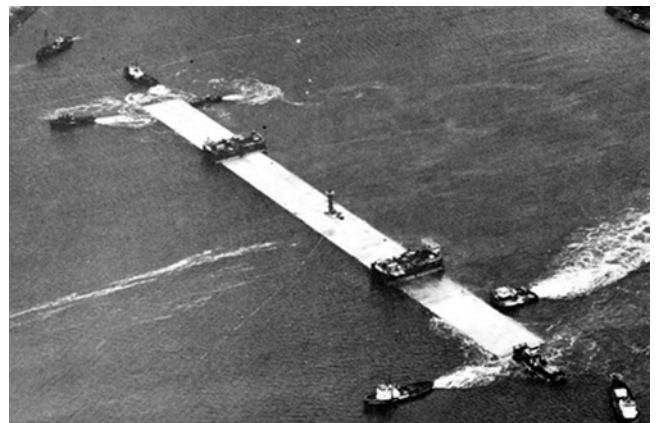
Fig. 3.16—Tunnel elements being towed into position.
