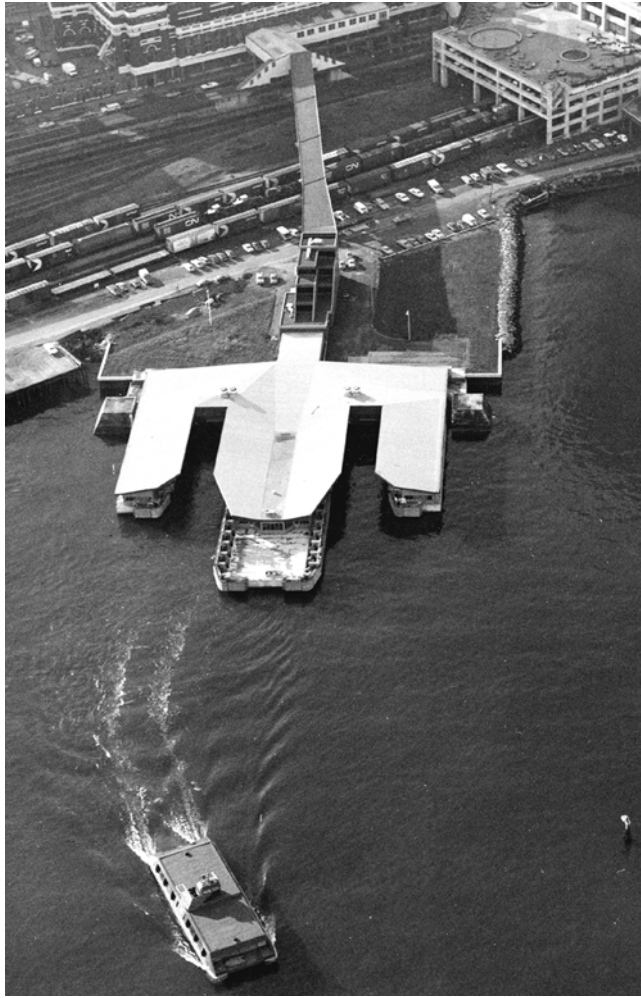
Fig. 3.9—Concrete floating dock, Vancouver, BC, Canada.
