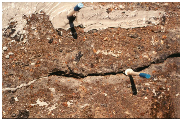
Fig. 3—Crack repair by epoxy pressure injection.
