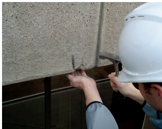
Fig. 3.3—Localized sampling during a preliminary assessment (photo courtesy of Wiss, Janney, Elstner Associates, Inc.).
