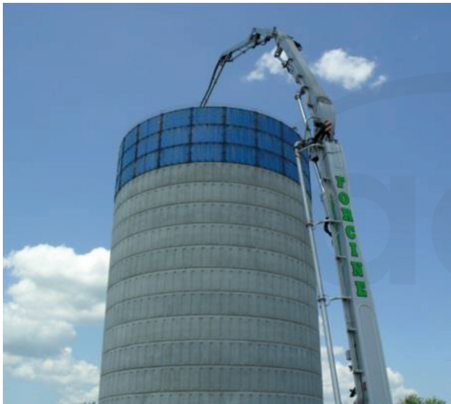
Fig. 1.4g—Construction of composite elevated tank pedestal (photo courtesy of Caldwell Tanks, Inc.).
