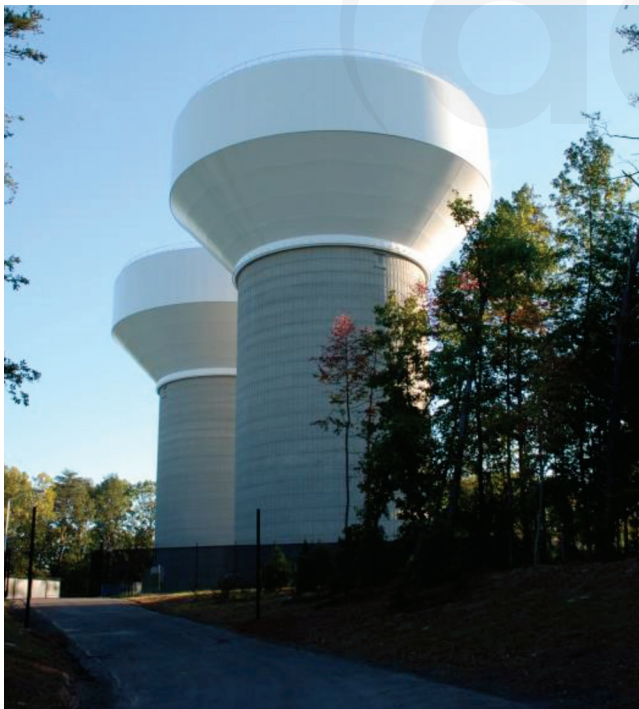
Fig. 1.4c—Completed composite elevated tanks (photo courtesy of Caldwell Tanks, Inc.).
