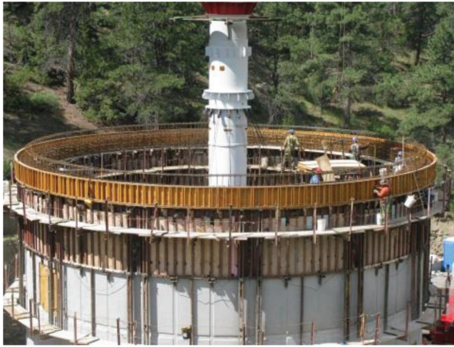
Fig. 1.4f—Construction of composite elevated tank pedestal (photo courtesy of CBI).
