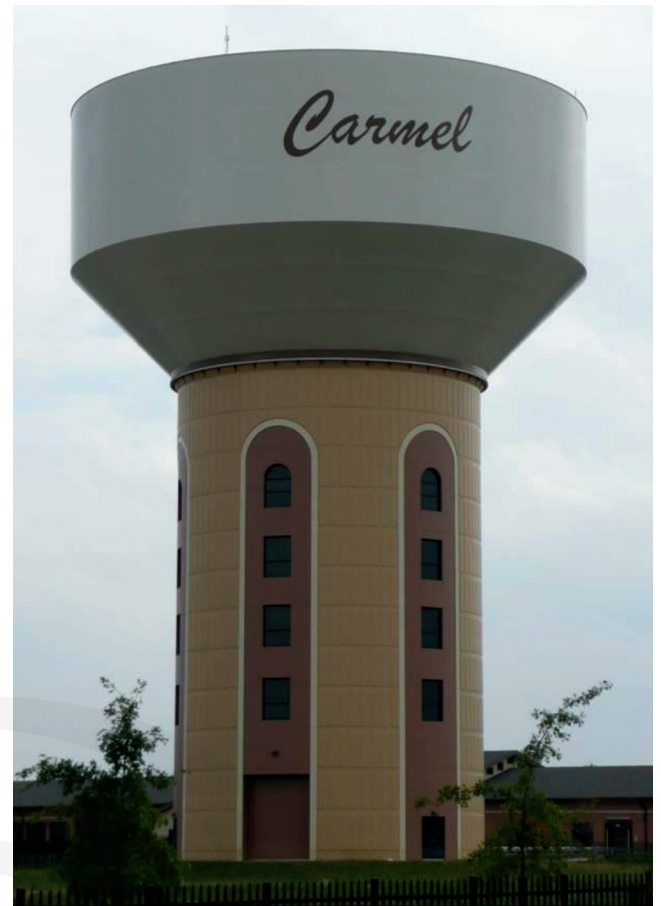
Fig. 1.4a—Completed composite elevated tank (photo courtesy of Landmark).
