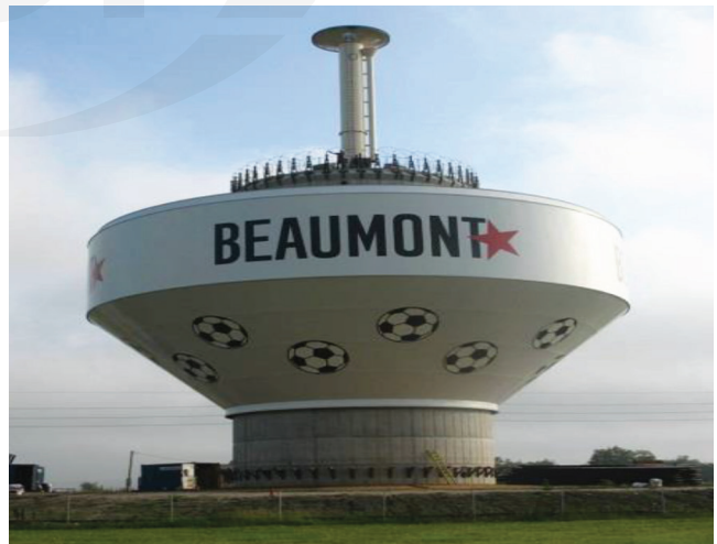
Fig. 1.4e—Construction of composite elevated tank (photo courtesy of Landmark).
