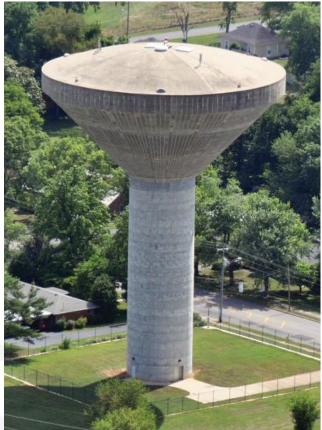
Fig. 1.4d—Completed concrete elevated tank (photo courtesy of Crom LLC).
