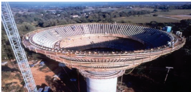
Fig. 1.4h—Construction of concrete elevated tank (photo courtesy of Crom LLC).
