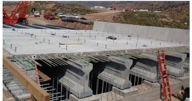
Fig. 3.2d—Emma Park Bridge deck panel with GFRP reinforcing bars, top and bottom mat.
