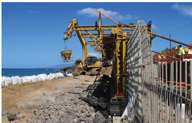
Fig. 3.2f—Construction of seawall with GFRP bars.
