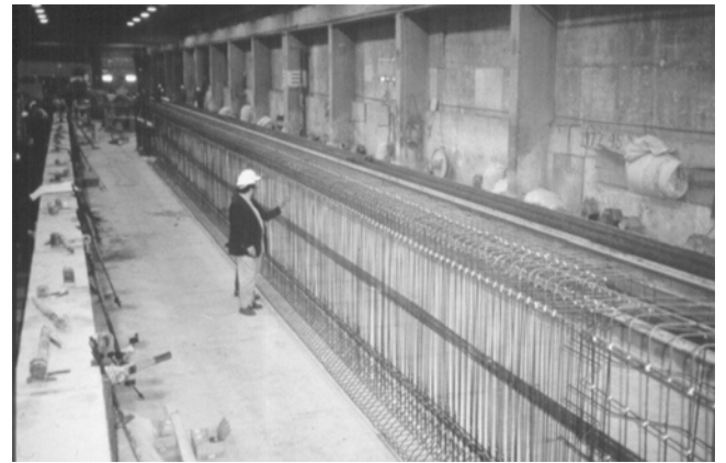
Fig. 1.2—Construction of the FRP prestressed girders for the Taylor Bridge in Headingly, Manitoba, Canada.
