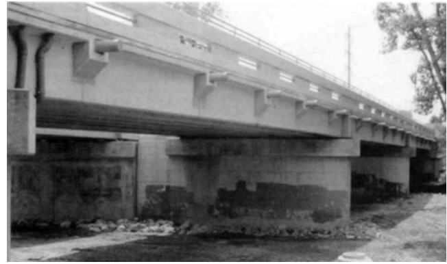
Fig. 1.5—Completed Bridge Street Bridge (Grace et al. 2002).
