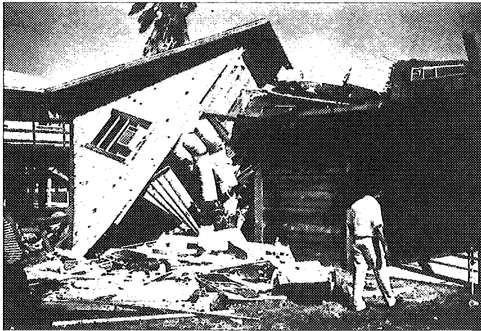
Fig. 1.3.1(a)—Typical damage to weak construction from hurricane winds
