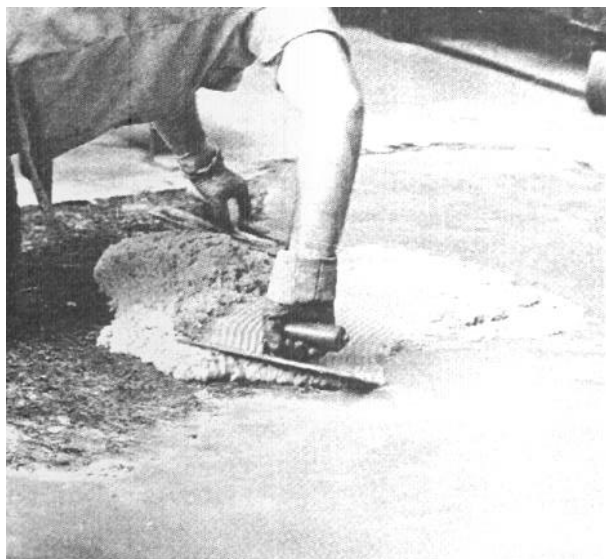
Fig. 4.1 -- Application of a thin epoxy mortar floor coating in an area subject to abrasion and chemical attack (courtesy Sika Chemical Corp.)
