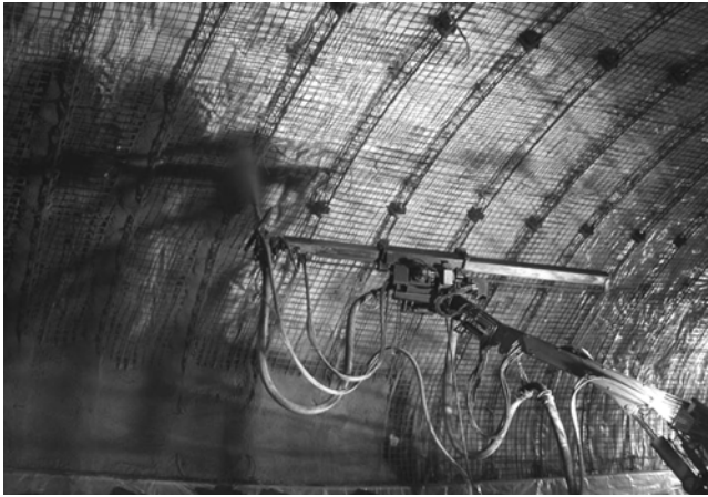
Fig. 5.9—Typical lattice girder during shooting (robotic).
