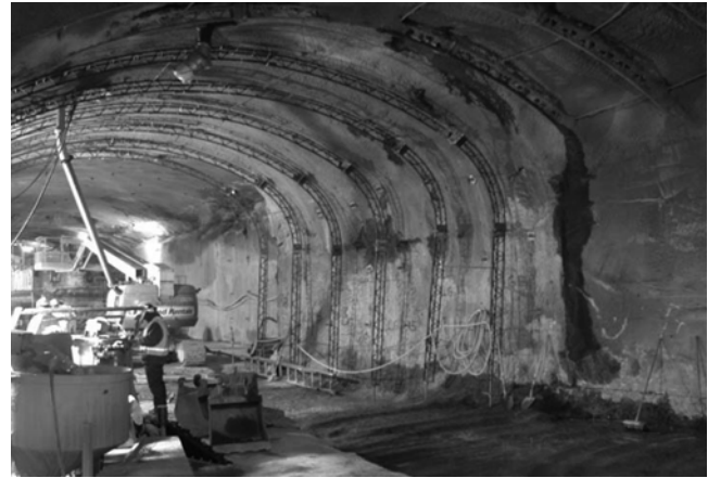
Fig. 5.11—Tunnel with lattice girders.
