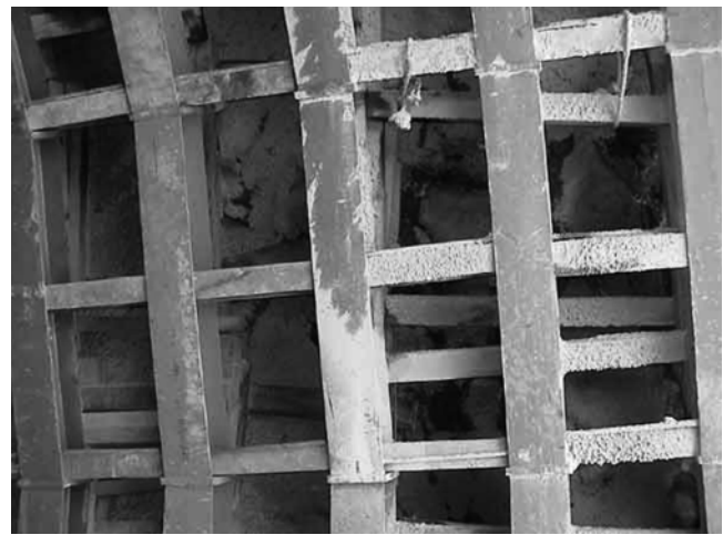
Fig. 5.12—Steel sets with significant wood cribbing.
