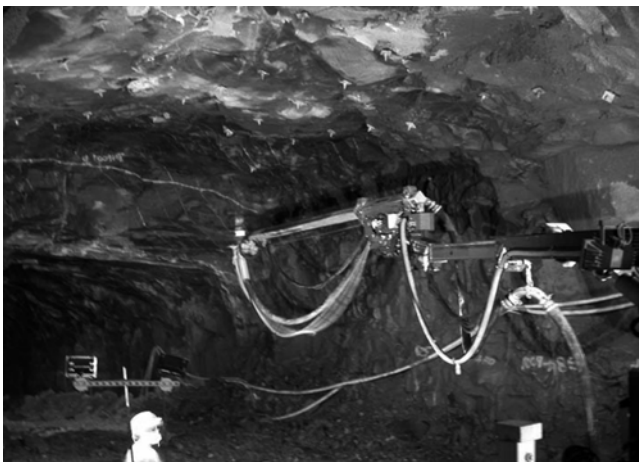
Fig. 5.3—Tunnel with pattern bolting before shotcreting.
