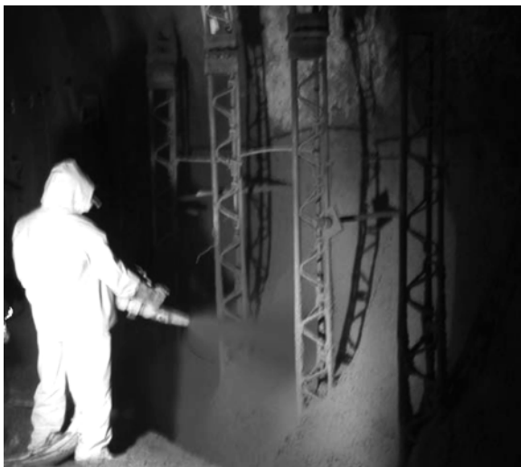
Fig. 5.10—Typical lattice girder during shooting (manual).
