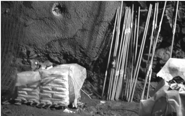
Fig. 5.2—Rock bolts and grout.
