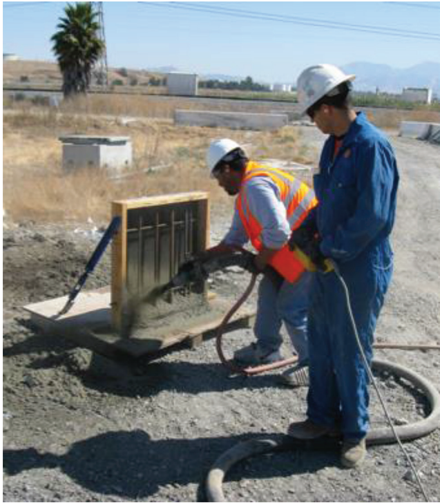
Fig. 1.6.3.1.2—Shooting certification panel with reinforcement.
