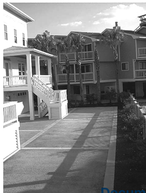
Fig. 3.1—Parking lot built with pervious concrete pavement
