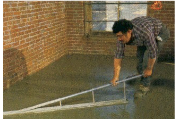
Fig. 5.2—Finishing a cellular concrete floor.
