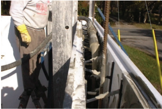
Fig. 5.1.1—Reusable formwork for a wall panel
