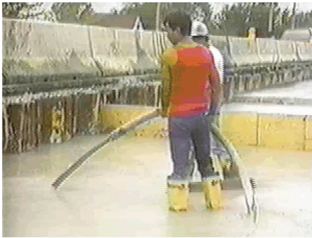
Fig. 5.1.2—Flowability of cellular concrete (video courtesy of Elastizell). See related video at http://www.concrete.org/Portals/0/Files/Media/ACI_523.3_Figure_5.1.2_Self-Leveling.mp4
