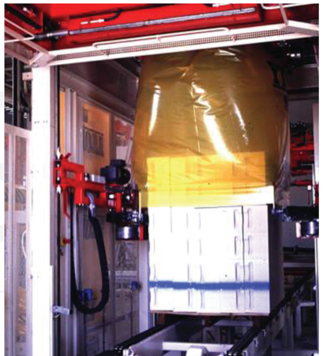
Fig. 3.4.4b—Packaging of finished AAC units.
