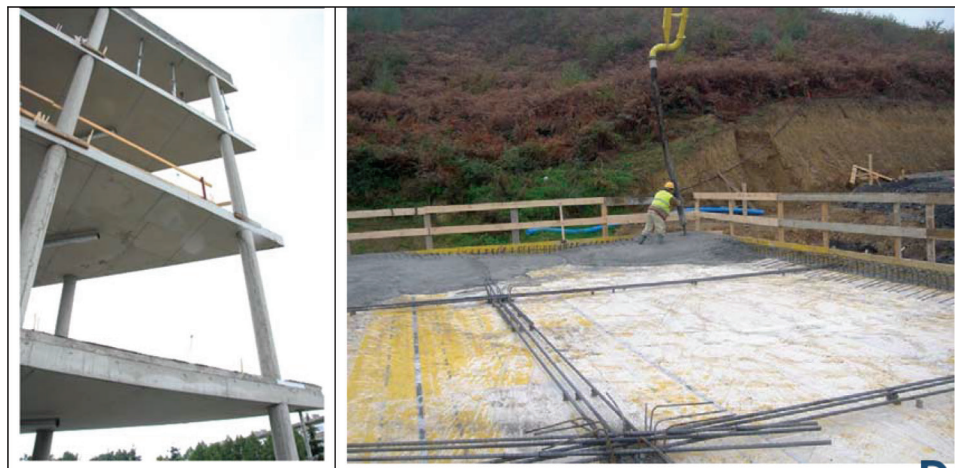
Fig. 1.1b—Construction and applications of E-SFRC slabs (courtesy of Primerks SIA) Document Sharing Hub
