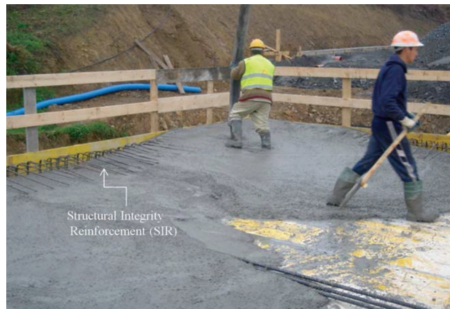
Fig. 4.4.1a—Casting of E-SFRC slabs using SFRC.
