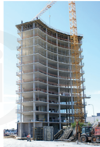
Fig. 4.3—Construction of multi-story elevated slab for residential/office building (Destrée and Mandl 2008).
