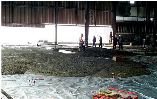
Fig. 1.1a—Installation of G-SFRC slab (pile-supported ground slab) (courtesy of Bombardier Aerospace Inc.).
