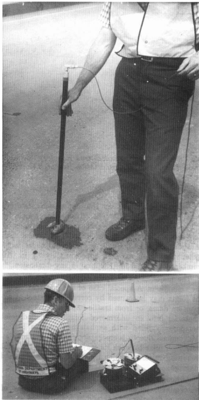
Fig. 2 – Corrosion detector (courtesy Federal Highway Administration).
